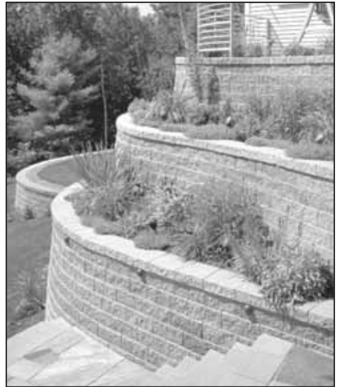
Tiered walls with plantings provide an attractive alternative to a single tall wall.
