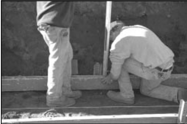
1. Set and level metal screed forms.
