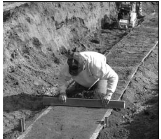
5. Screed sand for final leveling of pad.
