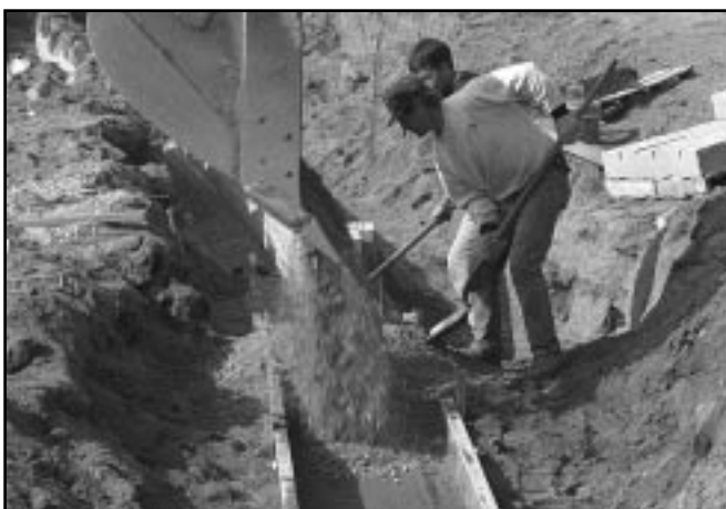
3. Fill forms with granular base material.
