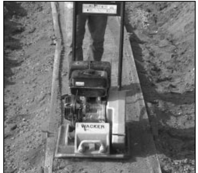
4. Compact leveling pad granular material.
