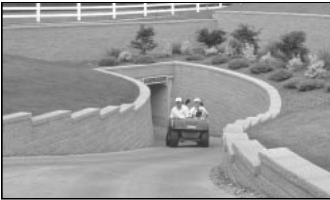
VERSA-LOK® cap units help create an "eyebrow" effect on the top of walls.
