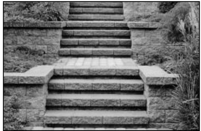
Often, stairs are built into retaining walls, inset between sidewalls.
